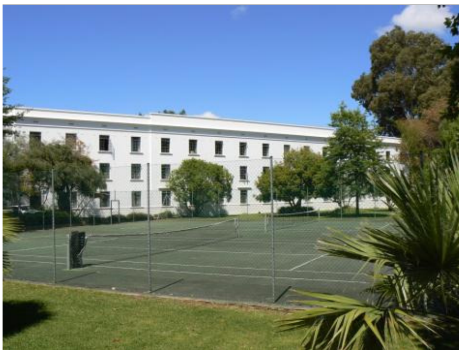
FIGURE 26: View of the tennis courts from Victoria Street with the Main Residence in the background (RC de Jong 24.11.2011)
