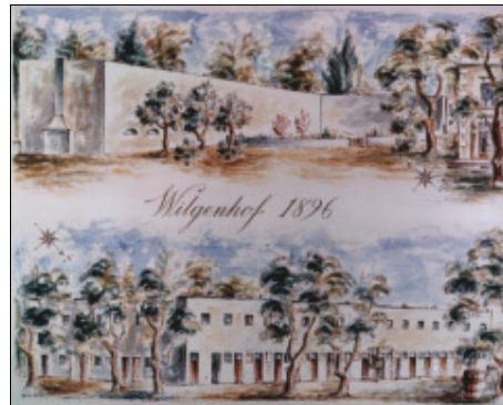
FIGURE 38: Artist's reconstruction of the farmstead in 1896 (two views) showing the L-shaped service buildings after the Louws had added a top storey. Bachelors is to the extreme top right. (Wilgenhof Archives)
