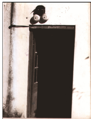
FIGURE 30: Historical photo of telephone building – note the external ringer (Wilgenhof Archives)
