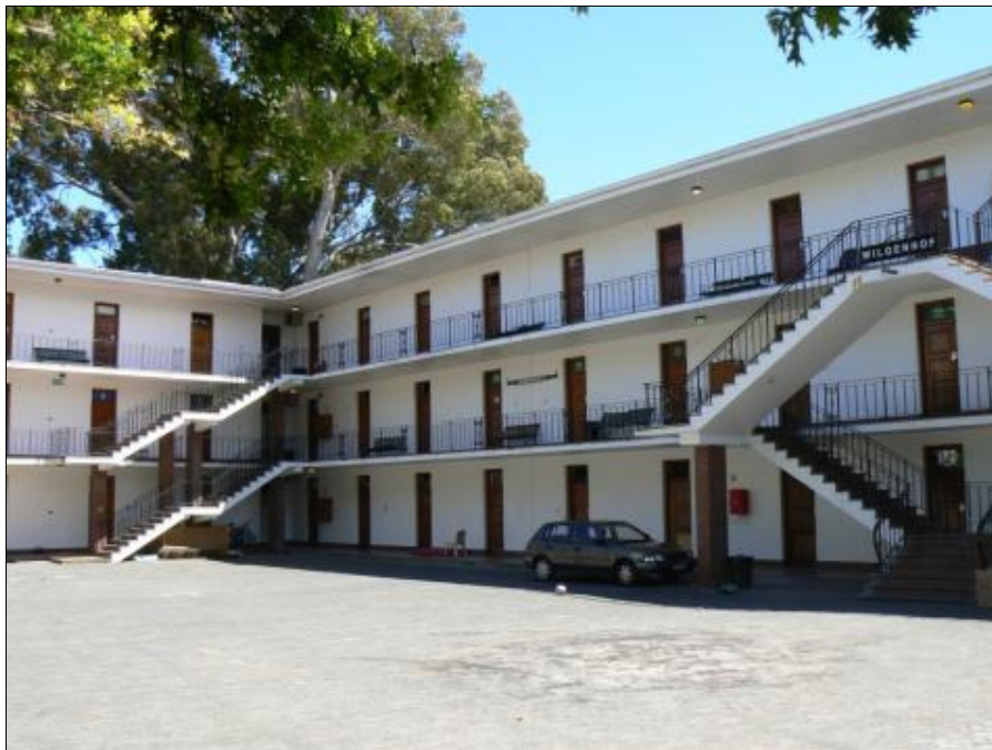
FIGURE 7: Courtyard with main staircase (V-Trap) on the right (RC de Jong 24.11.2011)
