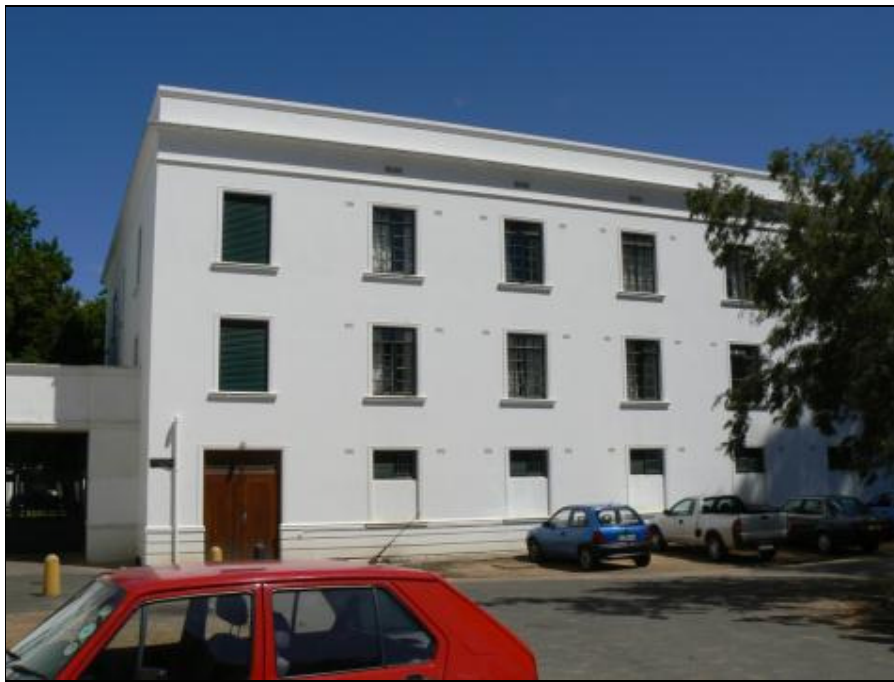
FIGURE 6: View of east façade (RC de Jong 24.11.2011)
