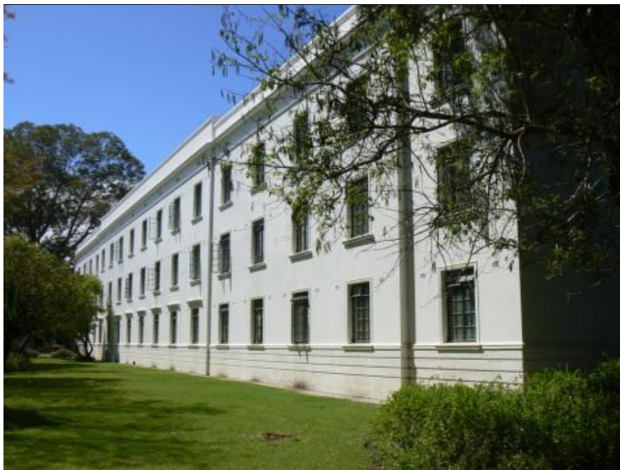
FIGURE 25: Portion of the garden between Main Residence and Victoria Street (RC de Jong 24.11.2011)
