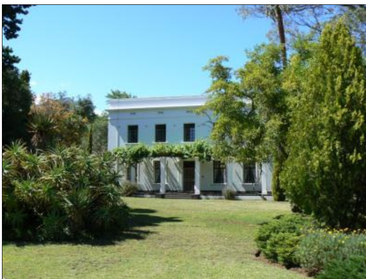
FIGURE 31: Main (north) façade, Hamelhof (RC de Jong 24.11.2011)
