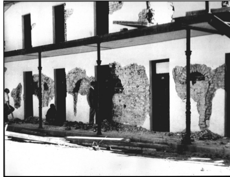
FIGURE 49: Hidden elements of the original farm outbuildings, such as these semi-circular windows, were revealed during its demolition in 1963 (Wilgenhof Archives). It is not yet known how well this demolition process was documented.
