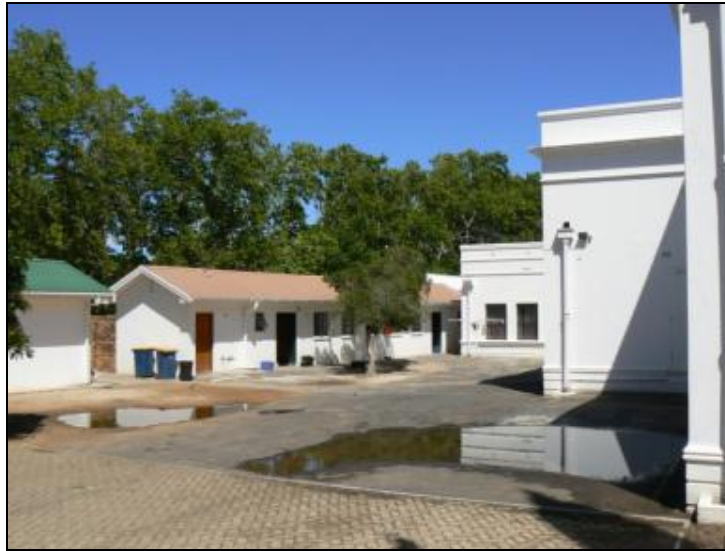
FIGURE 18: General view of the service yard with service buildings (left) and Wilgenhof Wing (right) (RC de Jong 24.11.2011)
