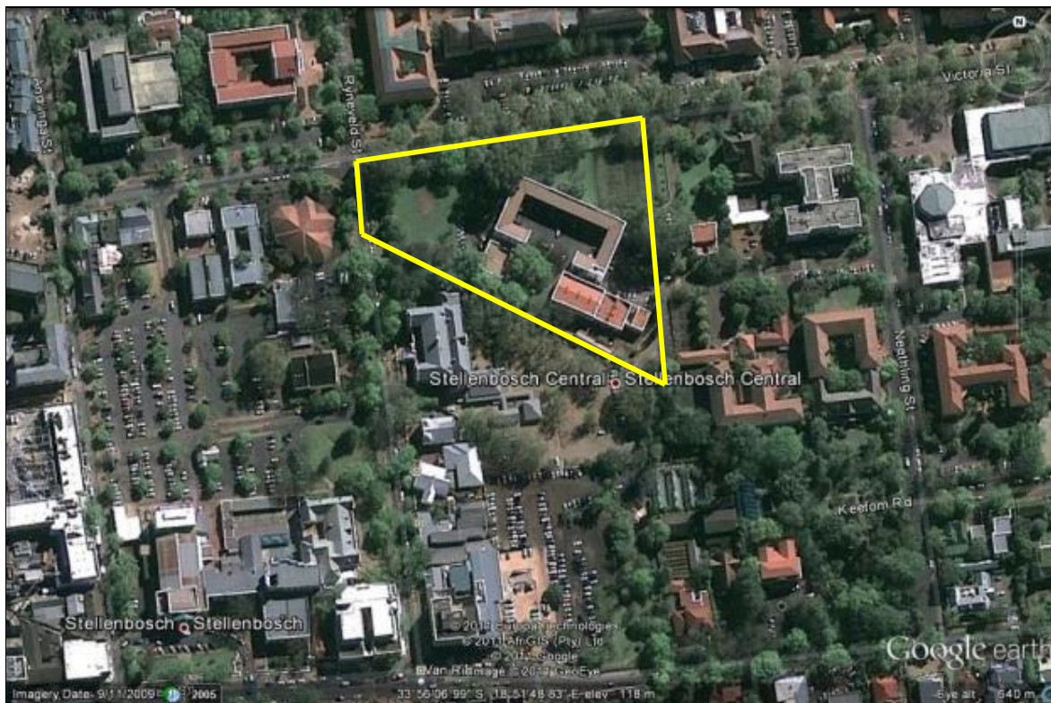
FIGURE 3: Google Earth image (2009) indicating the location and boundaries of the Wilgenhof site
