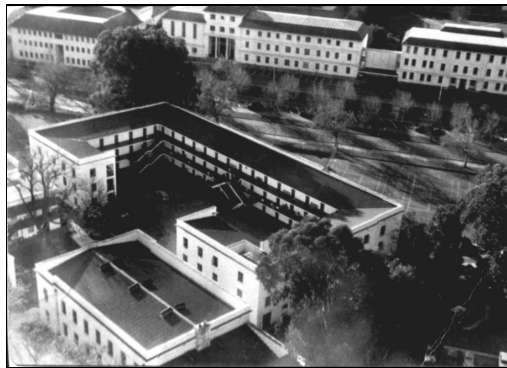
FIGURE 48: Aerial view of the Wilgenhof complex (Main Residence, Bachelors and Wing) taken shortly after the completion of the Wilgenhof Wing in the mid-1960s (Wilgenhof Archives)
