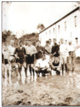
FIGURE 40: Construction of the tennis courts, 1906 (Wilgenhof Archives)
