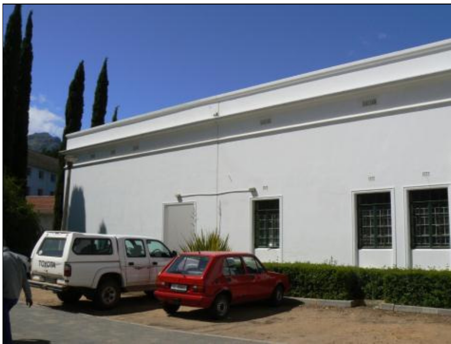
FIGURE 14: North façade of wing with kitchen section (right) and squash court (left) (RC de Jong 24.11.2011)
