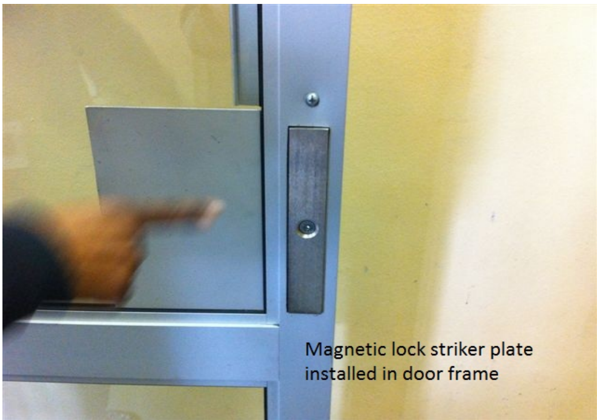
Magnetic Lock on Single Aluminium Door with Magnetic Lock Recessed in Stationary Post and Magnetic Lock Plate Recessed in Door 1.3.6
